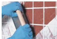
ARDEX WA: Excess Removal
