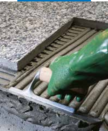
External installation of relief terrazzo "graniglie" tiles
