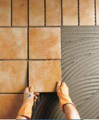
External installation of klinker tiles
