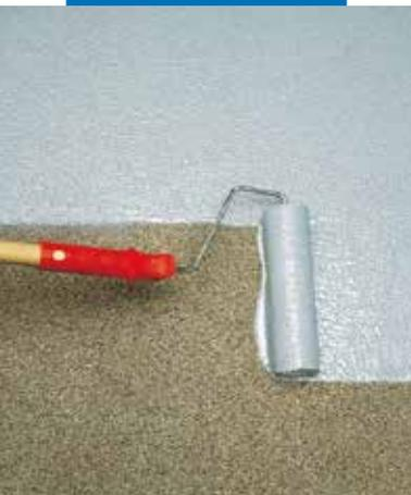
Applying Mapecoat I 24 with roller
