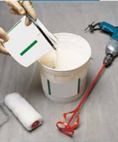
Mixing component B with component A
