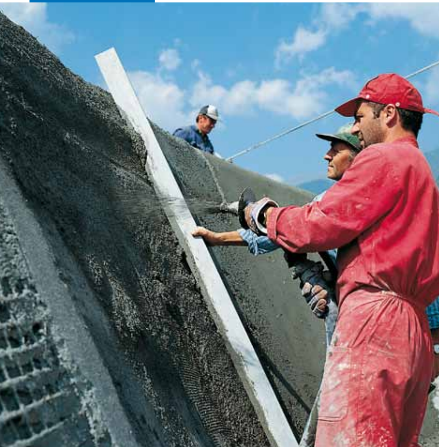
Spray application of Mapegrout T40
