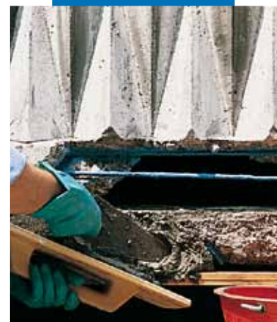
Repairing a balcony with Mapegrout T40
