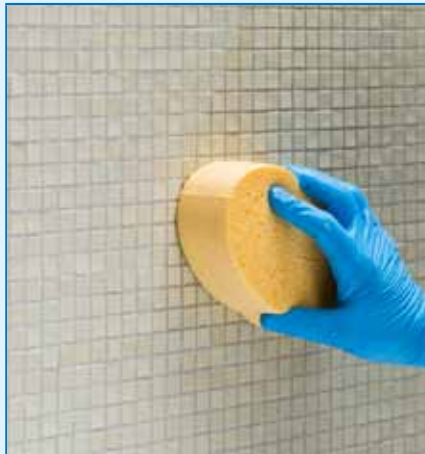
Cleaning and finishing the joints with a hard cellulose sponge
