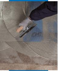
Placing Mapenet 150 on the first layer of Mapelastic Turbo while wet
