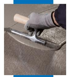
The second layer of Mapelastic Turbo over the first layer reinforced with Mapetex Sel
