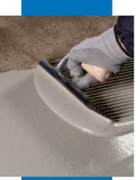
Application of the first layer of Mapelastic Turbo
