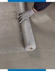
Placing Mapenet Sel on the first layer of Mapelastic Turbo while wet
