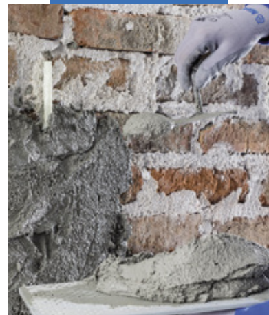
Application of the first layer of MapeWall Render & Strengthen
