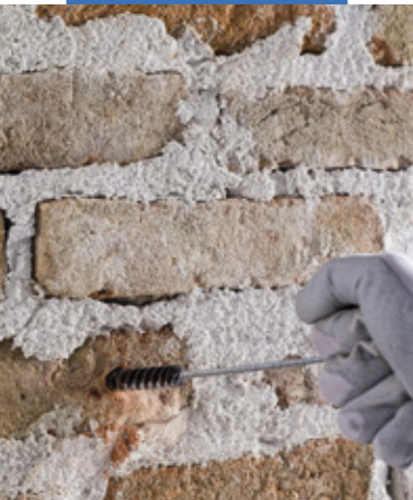
Removing dust from the holes
