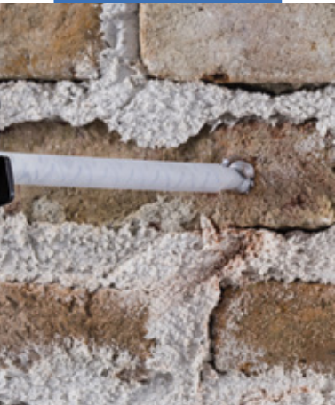
Application of the chemical anchor
