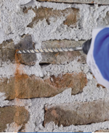
Drilling the holes
