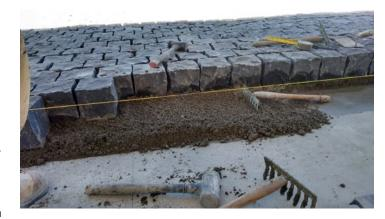
The resulting mixes have good freeze-thaw stability and are resistant to oil and many chemical environments. Placement thickness may be in the nominal range 40mm to 75mm in a single layer.
