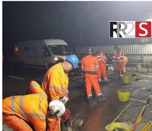
When used with a low water content, Patchroc 250 is designed for horizontal use, though it can be applied at gradients up to 2.5%.
