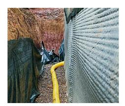
Platon DOUBLE DRAIN must be installed over a primary membrane, such as brushed on bitumen coatings. Fix Platon DOUBLE DRAIN along the top edge above the primary membrane, with Platon DOUBLE DRAIN cramps at 250mm centres. Overlap vertical joints by 500mm and horizontal joints by 150mm. Filter fabric can be pulled back for successive overlap of the membrane and filter fabric.
