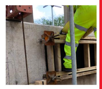
generally up to 150 mm thick although greater thicknesses may be achievable dependent on the configuration of the repair location and the volume of exposed reinforcing steel. Consult the local Fosroc office for further information.
