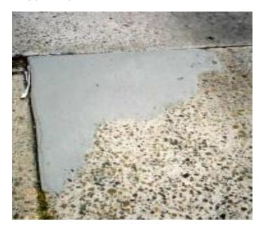
TamCrete Bond & Seal is a formulated acrylic admixture used both as a primer for wet-to-dry cementitious systems and as an emulsion in mixtures.
