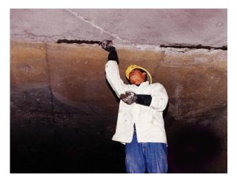
TamCrete Plug is a fast setting, hydraulic compound that instantly stops running water or seepage through masonry surfaces. It becomes harder and more resistant when subjected to moisture. TamCrete Plug is a non-shrink material that expands slightly and sets in about 70 seconds depending on the temperature of the mixing water and the surface to which it is applied. Lower temperatures will retard the set time; higher temperatures will accelerate the set time.
