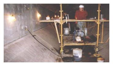
TamPur 170 is based on a prepolymer of polyurethane (Part A) and a polyol component (Part B). The product has been formulated to reduce foaming during the reaction with the polyurethane prepolymer, giving a hydrophobic injection resin. The non-toxic plasticizer is used so the cured resin is eco-friendly.
