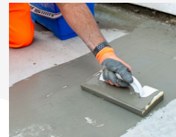
Brush apply tuffbond to the base* and to the underside of the paving units
