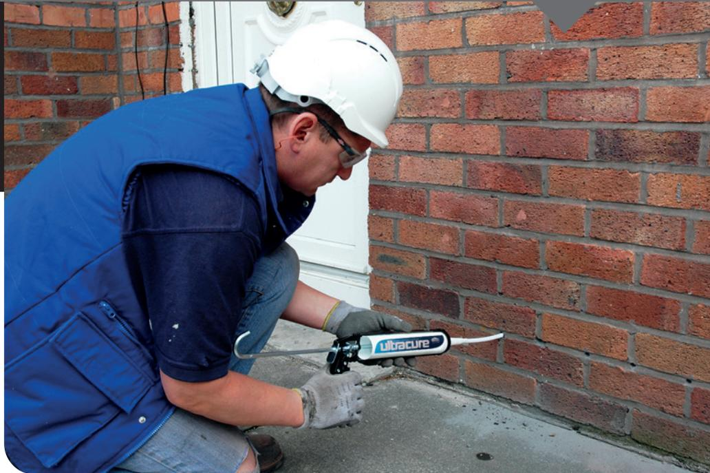
The cream is delivered by hand pressure from the appropriately sized applicator gun into a series of holes drilled into the mortar course.
