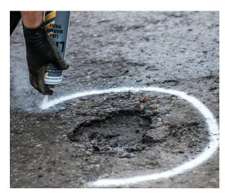
Ideal as an effective and quick method for line or spot marking of pothole repairs, car parks, warehouses, sports halls and building sites.
