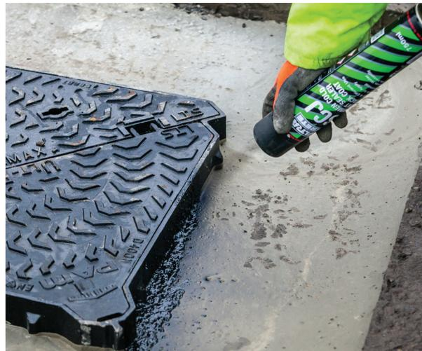
A cold joint sealer that is applied onto vertical edges and surface base before the application of asphalt.
