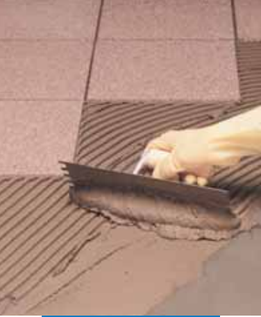
Example of porcelain gres laid on Mapelastac using Ultraflex S2 Quick
