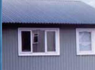
Metal roofing panels, coated with standard grey colour METAL-KOTE.
