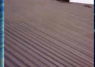
METAL-KOTE colour matched to original plastic coated profile metal roofs. which were flaking and peeling.
