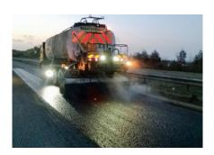
Colbond Multi is a polymer modified cationic bitumen emulsion designed to be applied both as a bond coat and vertical joint paint. Colbond Multi forms a uniform film of polymer modified bitumen on both horizontal and vertical faces forming a strong adhesive bond between bituminous overlay and the existing surface. In addition the application of it also improves the waterproofing of the road pavement. Colbond Multi, when fully broken, prevents 'pick-up' on the wheels, tracks or tyres of the
