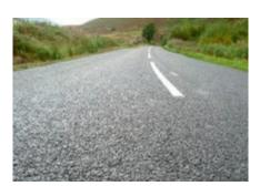
Secure Chip is a spray applied emulsion binder for application to recently completed surface dressings. It is a designed to reduce the amount of post sweeping required by securing the dressing aggregate in the mosaic structure minimising the risk of damaged windscreens from chippings dislodged by passing vehicles. Application of Colas Secure Chip also gives a pleasing aesthetic and long lasting black colour resembling an asphalt surface.
