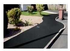
Cationic Slurry Seal Emulsion (CSS) is a key constituent of slurry seal for hand or machine application. Ideal for rejuvenating cracked, spalled and worn surfaces, it is based on a K3 cold emulsion with a fast application and drying time of approximately 30 minutes. This means that the material can be laid quickly, economically and safely with the minimum disruption to road users and residents.
