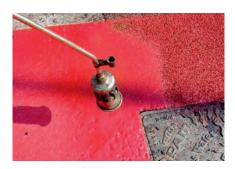
Antiskid Sheets are skid resistant thermoplastic sheets available in a variety of colours which are ideal for application on bus and cycle lanes as well as other high stress areas. They are easy to use, can be cut to size and are instantly trafficked once cooled. **Antiskid Sheets** are non-toxic, contain no lead or chromate pigments and are skid resistant to >55 SRV.
