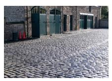
Sett Grout is a hot applied bituminous compound which secures all types of setts/cobbles. It has been developed in order to solve the pouring and setting problems encountered with some filled bitumen grouting materials. Adhesion, flow and pouring properties have been improved whilst still retaining recommended softening point and penetration characteristics.
