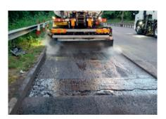
**Colbond 50** is nominally a 50% binder content polymer modified bitumen emulsion. It forms a uniform film of polymer modified bitumen on the road surface which promotes a strong adhesive bond between a bituminous overlay and the existing surface. The application of **Colbond 50** also improves the waterproofing of the road pavement.
