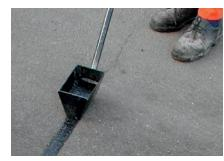
Jointgrip OB is an anti-skid overbanding joint sealant. It is a proprietary formulation of blended paving grade bitumen incorporating special polymers and abrasive aggregates to provide a compound of toughness, flexibility, adhesiveness and resistance to flow.
