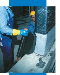
Application of MapeWrap onto the reinforced concrete element to saturate the fabric and remove the excess resin.
