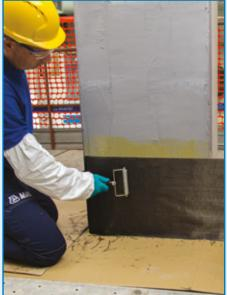
Application of MapeWrap C UNI-AX fibre impregnated with MapeWrap 31
