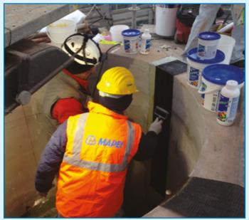
Brickwork chimney strengthened with the MapeWrap C UNI-AX System
