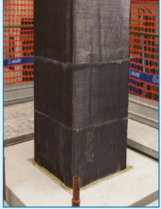
Pillar confined with the MapeWrap C UNI-AX System
