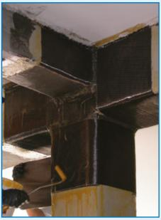
Beam-pillar joints confined with the MapeWrap C UNI-AX System
