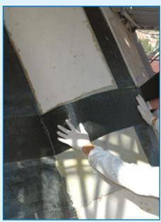
Domed roof strengthened with the MapeWrap C UNI-AX System
