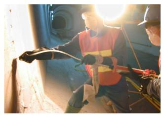
TamRez 210 is a low modulus, extra low viscosity, epoxy adhesive designed to be injected into cracks which exhibit minor movement or are subject to shock or vibration. Its low viscosity allows maximum penetration into small, hairline cracks or fractures. After injection and in its cured state, TamRez 210 returns structural integrity and protects reinforcement while at the same time compensating for minor movement and vibration.
