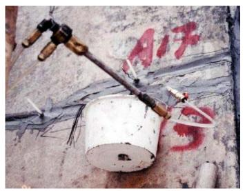
TamRez 220 is a high modulus, low viscosity, epoxy resin designed for injection into non-moving cracks in concrete structures. Its medium to low viscosity will allow maximum penetration into small cracks. TamRez 220 exhibits extremely high strength in its cured state, thereby restoring structural integrity. It is moisture insensitive, allowing for injection into damp cracks.
