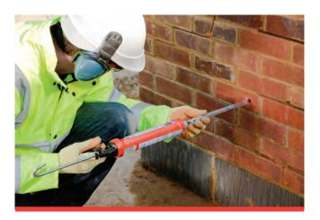
Injecting resin to complete the RetroTie installation
