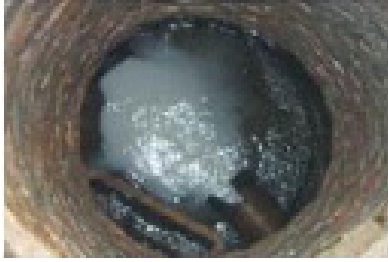
Mars, PA, Brick manhole
