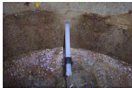
Insertion of static mixer at joint
