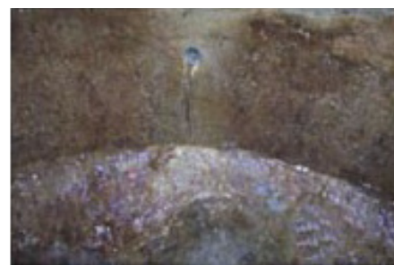
Results after drilling 16mm hole
