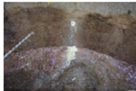
100% complete seal of joint 360° - 2 sets of SealGuard II
