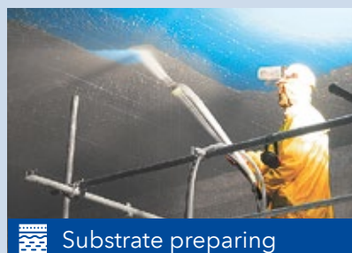
Spraying levelling mortar
