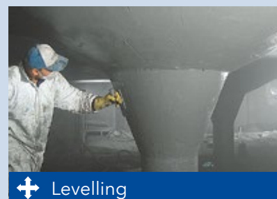
Spraying levelling mortar
