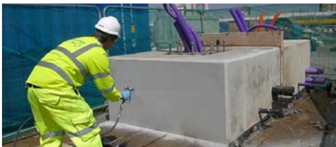
Cementitious Coating 851 effectively reinstates cover & protects from chlorides.
