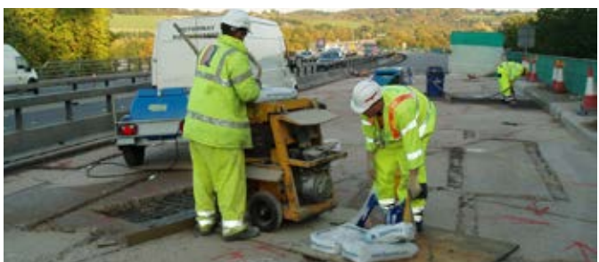
Fastfill sets in just 10 minutes & can achieve a final strength of over 60MPa.
