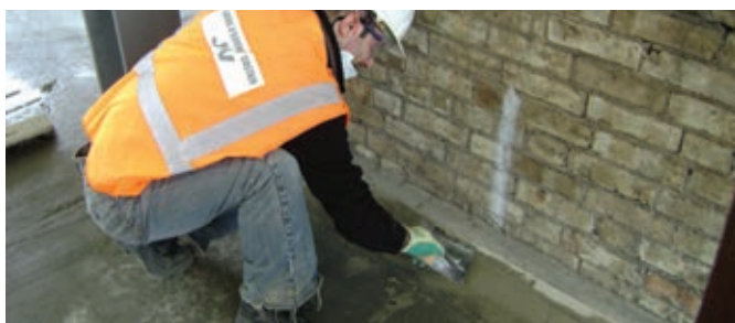
Monolevel RM is fibre-reinforced for added strength and durability.
