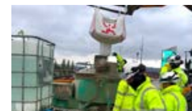
500kg bulk bags matching on site mixer capacity
