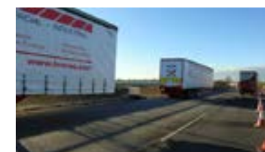
Supply direct to bridge deck
