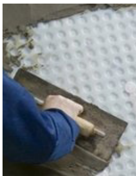
Proofex Cavitydrain PB - allows direct application of wet lining systems
