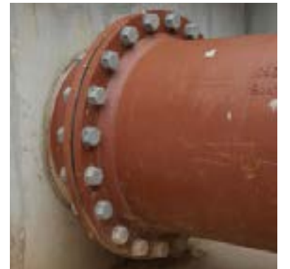
Grouting around pipe penetrations using Conbextra TS
