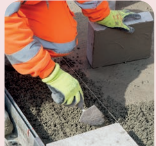
Step 6 Bed unit onto tuffbed mortar
