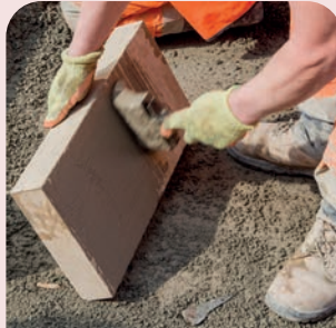
Step 5 Brush on the bonding mortar
