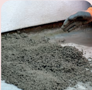
Step 4 Place tuffbed bedding mortar
